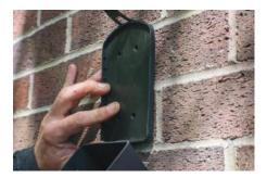
• Now use the 5mm drill bit to make a hole 55mm deep in each of the marked fixing holes
