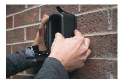
• Push the fixing bolts that have been supplied with your Keyguard XL into each of the holes
